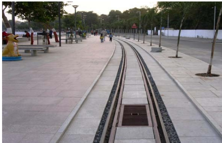
Fig. 19.24 Joy Train – Ballast - less Track at Kankaria Lake
