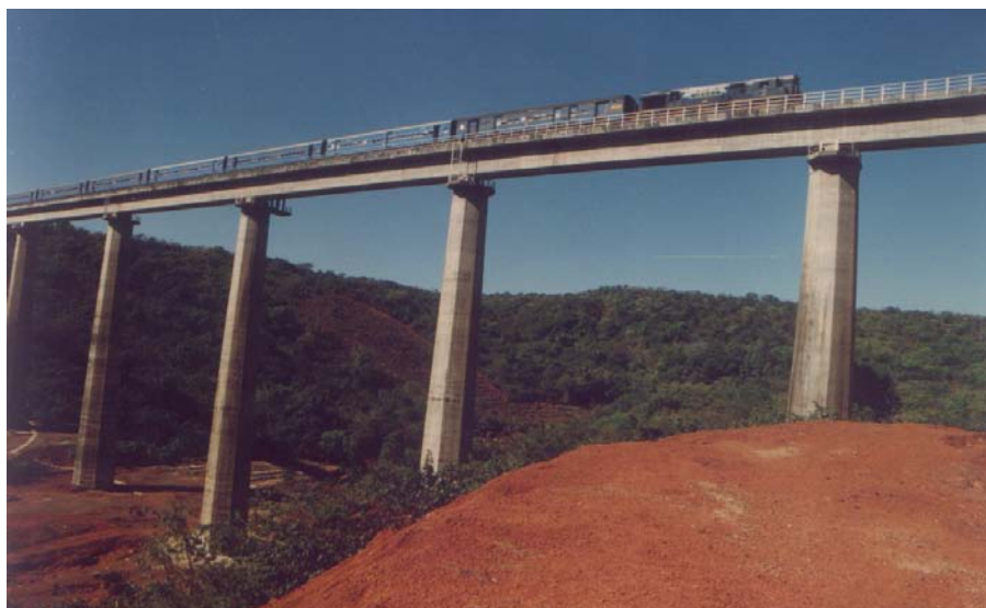
Fig. 19.13 Panval Nadi Viaduct
