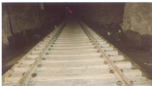
Fig. 19.18 Ballast - less Track in Long Tunnels
