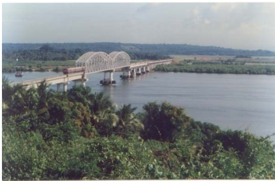
Fig. 19.14 Zuari Bridge – Goa
