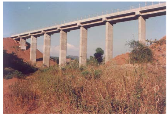
Fig. 19.9 RC Framed Viaduct
