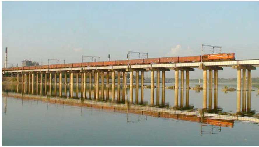
Fig. 19.1 Sabarmati Railway Bridge at Ahmedabad
