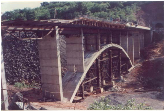
Fig. 19.8 Nandivli RC Arch Bridge
