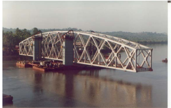
Fig. 19.15 Zuari Bridge – Launching
