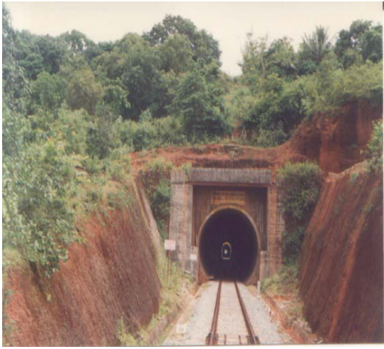
Fig. 19.16 Shield Tunnel at Honavar
