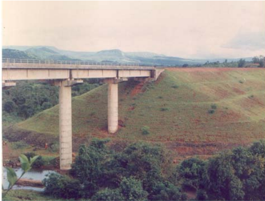
Fig. 19.4 Spill through Abutment
