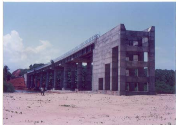
Fig. 19.5 3D RC Abutment
