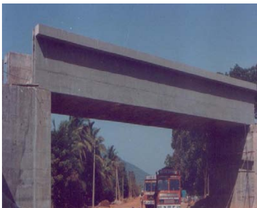
Fig. 19.10 PSC U Girder for a RUB
