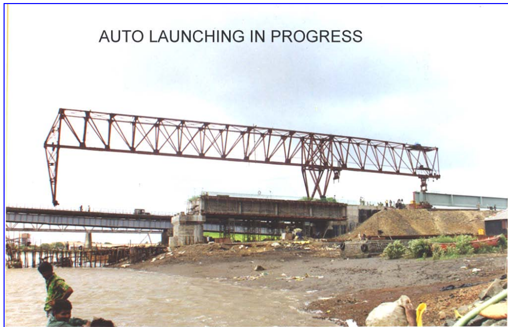
Fig 17.1 The launching girder
